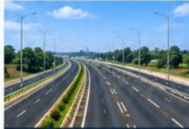
Road Construction & Rehabilitation Improving connectivity and economic growth.
