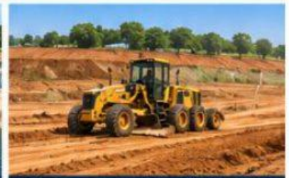
Site Development From earthworks to complete infrastructure.
