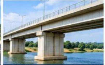
Bridge Construction Safe and durable structures.
